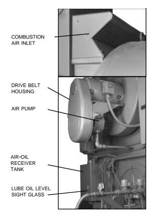
Figure: 2-21 Belt Driven Air Pump **Component Locations (CB)**
