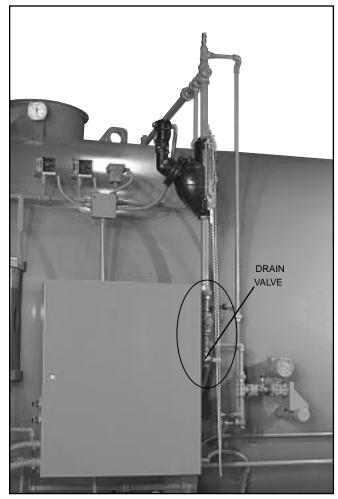
Figure: 1-6 Water Column Assembly
