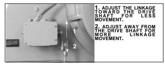
Figure: 6-3 Modulating Motor
