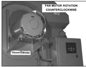
Figure: 5-1 Fan Motor CB-LE
