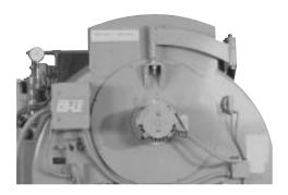
Figure: 2-7 Forced Draft Fan Motor CB-LE
