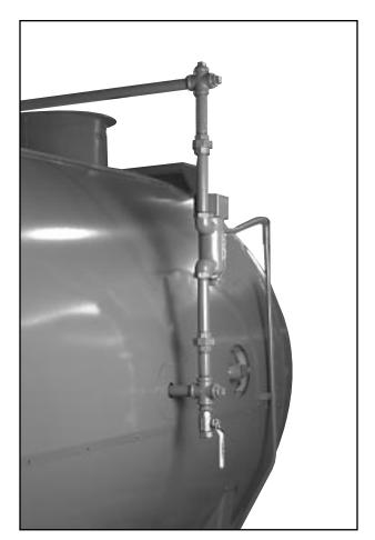
Figure: 1-8 Auxiliary Low Water Cut Off
