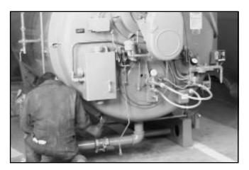
Figure 8-35: Close and Tighten Front Head
