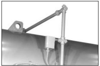
Figure: 1-13 Low Water Cutoff (LWCO Hot Water)
