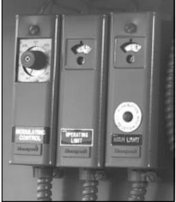
Figure: 6-5 Hot Water Controls
