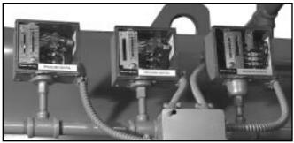
Figure: 6-4 Steam Operating Controls
