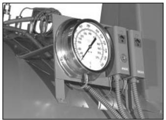
Figure: 1-11 Water Temperature Gauge
