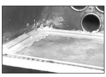
Figure 8-28: High Temperature Cement on Baffle Weld Area
