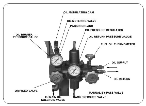
Figure: 2-18 Oil Control Valve Assembly -for Heavy Oil
