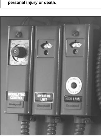
Figure: 1-12 Hot Water Controls
