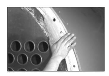
Figure 8-30: Apply Pulp Over Rope and Tadpole Gasket
