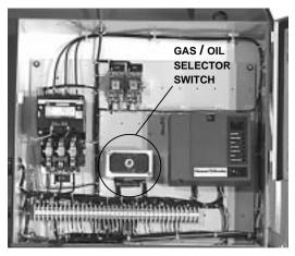
Figure: 2-23 Standard Control Panel
