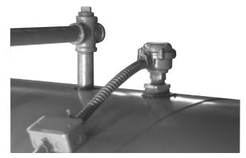
Figure: 1-14 Auxiliary Low-Water Cutoff
