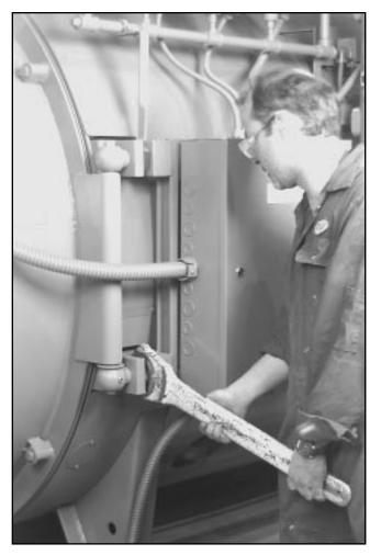
Figure 8-36: Tighten Hinge Bolts
