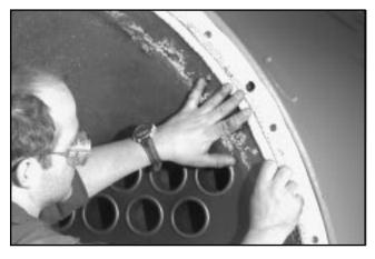
Figure 8-29: Rope Gasket Glued against Tadpole Gasket
