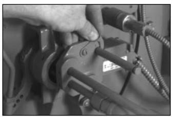
Figure: 5-9 Gun Locked In, Firing Oil
