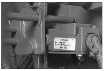
Figure: 5-10 Oil Drawer Switch Closed, Firing Oil
