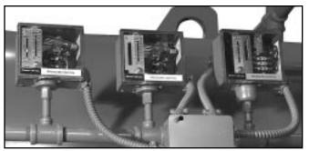
Figure: 6-7 Steam Operating Controls
